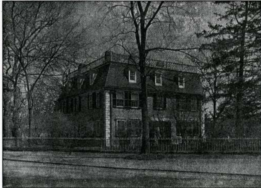
EDWARD EVERETT HOUSE used to stand at the corner of Boston Street and Columbia Road.
