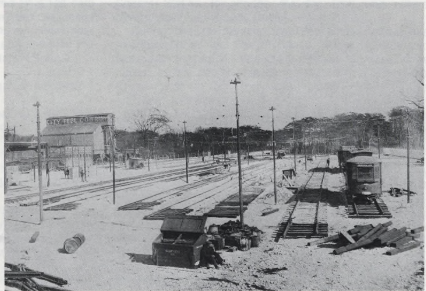
A second view taken the same day, October 28, 1929 showing track laying progress with compressor car #40 and a Type 2 car in use as a compressor in the rear.
