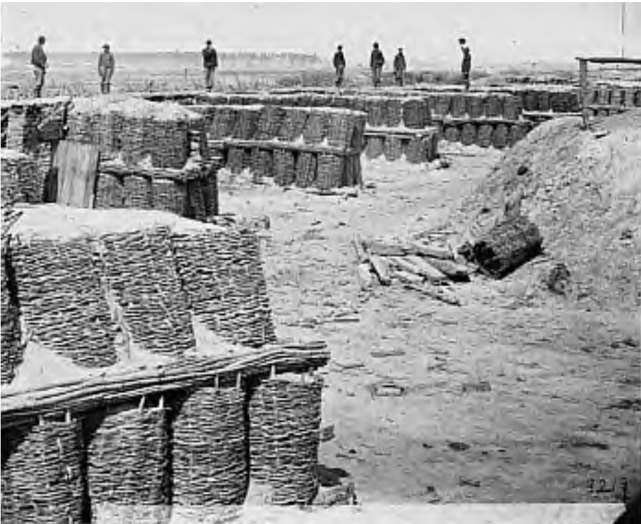
Gabions erected into walls and filled with earth in the Civil War
